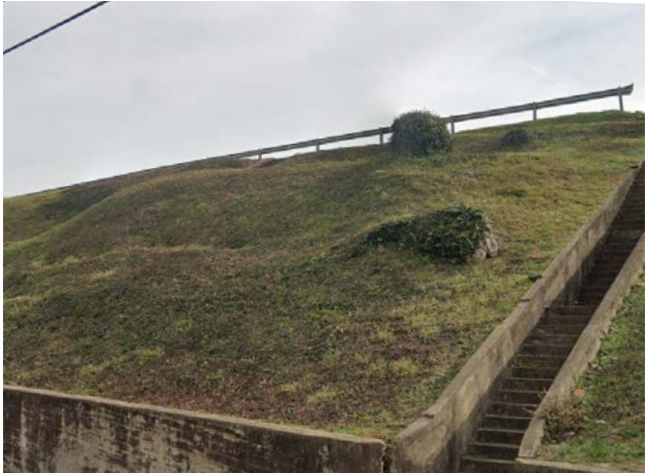
3. Existing Concrete Stairs along Sevier Ave.
