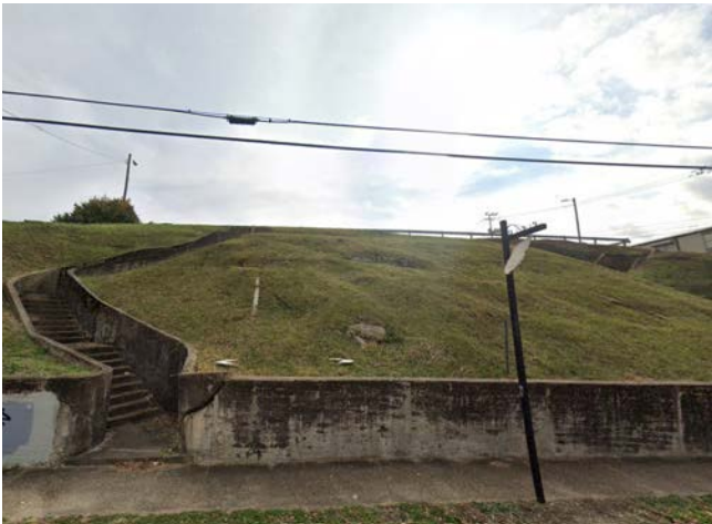
2. Existing Concrete Stairs along Sevier Ave.
