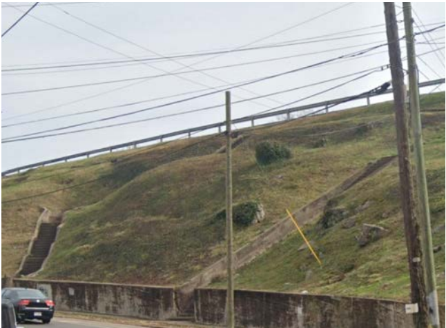
1. Existing Concrete Stairs along Sevier Ave.
